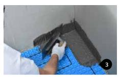
Apply the the same type of adhesive used for tiling to the corner (wall and floor) with a 3/16"X 3/16" (4 mm x 4 mm) notched trowel to a width of about 4" (100 mm).
