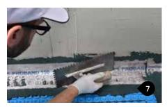
Using a flat trowel apply strong and even pressure along **PROBAND 150/250** to ensure sealing. Smooth over to avoiding and eliminate bends and folds.
