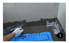
Apply the same type of adhesive used for tiling along the perimeter floor with the flat side of the trowel, to a width of about 4" (100 mm). Particular attention must be paid to fill the cavities of the Prodeso Heat membrane and leaving a thin layer of adhesive on top of the reliefs. Apply the same type of adhesive used for tiling to the perimeter wall with a  $3/16" \times 3/16"$  (4 mm x 4 mm) notched trowel to a width of about 4" (100 mm).
