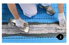
Fix **PROBAND 150/250** tape to the same type of adhesive used for tiling following the joint. Using a flat trowel apply strong and even pressure along **PROBAND 150/250** to ensure sealing. Smooth over to avoiding and eliminate bends and folds.
