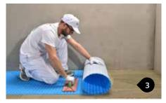
Press the membrane with a roller or a plastic flat trowel.
