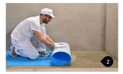
Apply **PRODESO HEAT MEMBRANE**, previously cut, on the adhesive.
