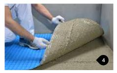
Check coverage of **PRODESO HEAT MEMBRANE**; in case of partial coverage, increase the amount of adhesive or its fluidity.
