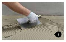
Attach a compatible adhesive to the substrate using a suitable trowel.
