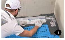
Fix **PROBAND 150/250** tape to the same type of adhesive used for tiling following the perimeter joint.
