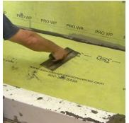
17. Carefully trim out the membrane covering the center flange recess with a sharp utility knife. Use the straight edge of a trowel to ensure that the membrane at the edge of the cut remains well bonded to the flange.
