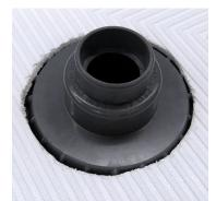
6. Test Fit drain flange directly to subfloor and measure distance to 2" diameter waste pipe fitting under subfloor. Cut and test the proper length coupler pipe that will attach flange to waste pipe but still allow the flange direct support at the subfloor. The top of the 2" pipe coupler should come to about 1-1/2" below the top of the subfloor (and sleeves inside drain outlet.) Ensure a successful dry fitting so that these will later glue together correctly
