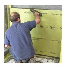
The remainder of the installation is going to follow this same sequence of installation procedures. For seamless continuation of the waterproofing, each new section will overlap the previous by 2 inches. The WP membrane features a dashed line near the edge as a guide to assist you in proper installation.
