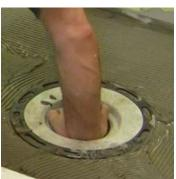
16. Now trowel out 3/16" notched modified thin-set mortar over the "fleece" region of the drain flange. However, DO NOT yet apply thin-set to the center pocket recess of the flange. Position, press in and set the floor piece(s) using the same installation techniques used previously.
