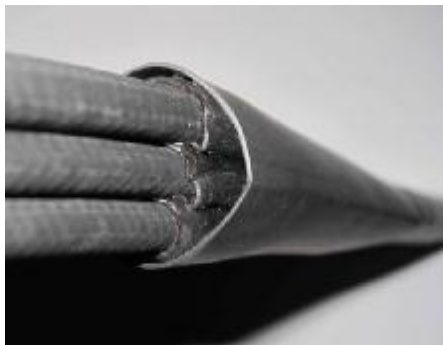
26. Slide the 203mm(8 inch)-long heat-shrinkable tube as shown.
