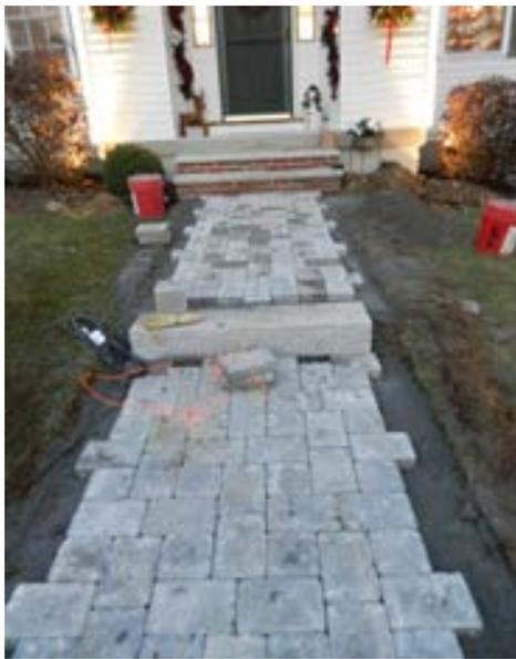
Although the granite surfacing where the heating mats were installed is approximately 7 inches thick, Tompkins found the product to be extremely efficient at melting the ice above when tested. For this reason, the system should serve as an adequate way to keep the driveway and walkway ice and snow-free in winters to come.
