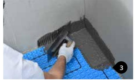
Apply the the same type of adhesive used for tiling to the corner (wall and floor) with a 3/16"X 3/16" (4 mm x 4 mm) notched trowel to a width of about 4" (100 mm).
