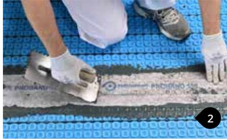
Fix **PROBAND 150/250** tape to the same type of adhesive used for tiling following the joint. Using a flat trowel apply strong and even pressure along **PROBAND 150/250** to ensure sealing. Smooth over to avoiding and eliminate bends and folds.
