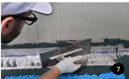
Using a flat trowel apply strong and even pressure along **PROBAND 150/250** to ensure sealing. Smooth over to avoiding and eliminate bends and folds.
