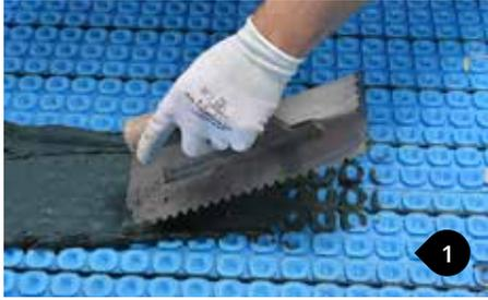
Apply the same type of adhesive used for tiling along the joints between two adjacent sheets with the flat side of the trowel, 4" (100 mm) each side of the joint), making sure to fill the cavities of the membrane, leaving a thin layer of adhesive on top of the reliefs.
