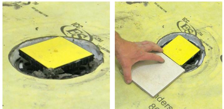
20. With a margin trowel or small flat blade, push high-quality modified thin-set mortar into pocket and into the locking grooves of the riser locking ring. This process will allow final adjustments while allowing a super solid, strong and well-supported riser and grate assembly after the thin-set has cured.
