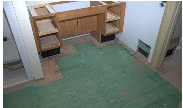
TempZone™ Installation for Bathroom 2
