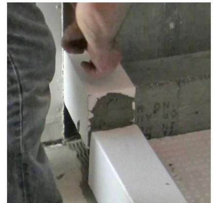
9. Dry fit your drain flange into the foam pocket and onto your plumbing 2" diameter waste pipe. The GEN II flange has locking grooves built into the bottom. Literally step on the drain flange to force the locking grooves into the foam pocket to guarantee a perfect seat for final installation. At this point, just leave the flange dry-fitted in place.
