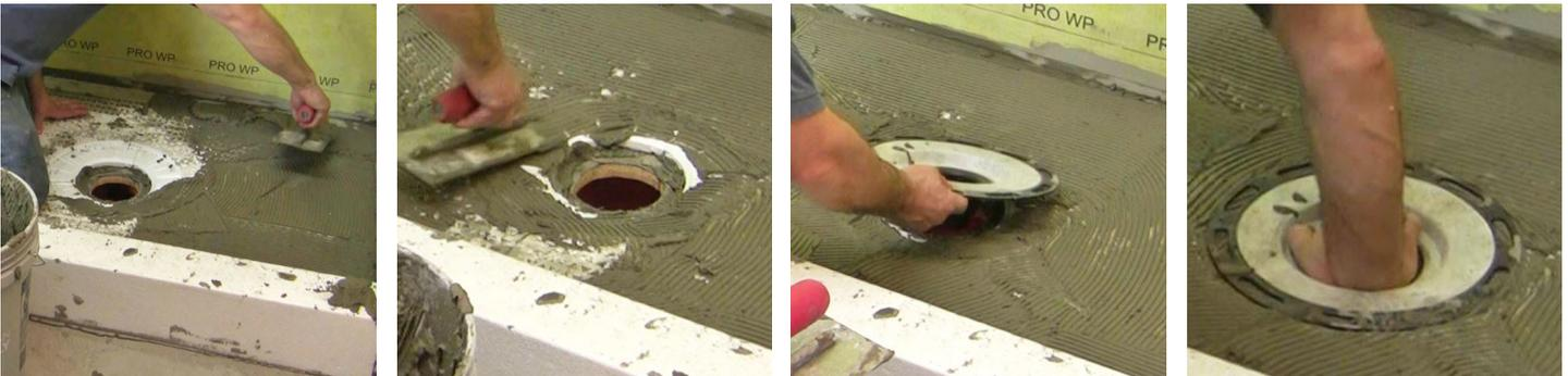
16. Now trowel out 3/16" notched modified thin-set mortar over the "fleece" region of the drain flange. However, DO NOT yet apply thin-set to the center pocket recess of the flange. Position, press in and set the floor piece(s) using the same installation techniques used previously.
