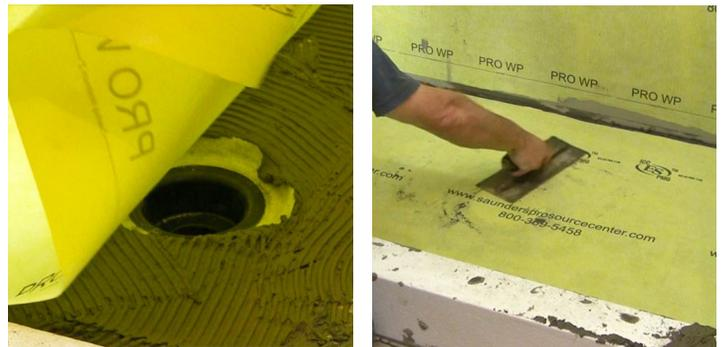
17. Carefully trim out the membrane covering the center flange recess with a sharp utility knife. Use the straight edge of a trowel to ensure that the membrane at the edge of the cut remains well bonded to the flange.
