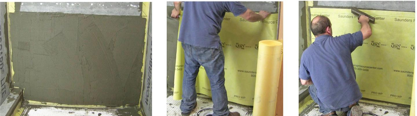
The remainder of the installation is going to follow this same sequence of installation procedures. For seamless continuation of the waterproofing, each new section will overlap the previous by 2 inches. The WP membrane features a dashed line near the edge as a guide to assist you in proper installation.
