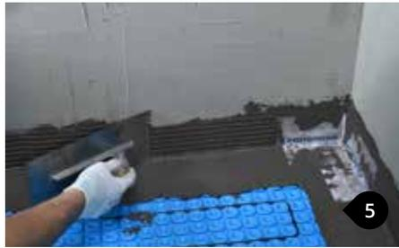
Apply the same type of adhesive used for tiling along the perimeter floor with the flat side of the trowel, to a width of about 4" (100 mm). Particular attention must be paid to fill the cavities of the Prodeso Heat membrane and leaving a thin layer of adhesive on top of the reliefs. Apply the same type of adhesive used for tiling to the perimeter wall with a 3/16" x 3/16" (4 mm x 4 mm ) notched trowel to a width of about 4" (100 mm).
