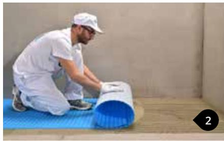
Apply **PRODESO HEAT MEMBRANE**, previously cut, on the adhesive.
