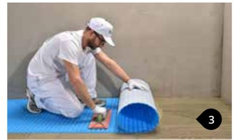
Press the membrane with a roller or a plastic flat trowel.
