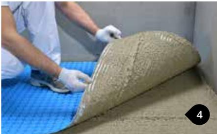
Check coverage of **PRODESO HEAT MEMBRANE**; in case of partial coverage, increase the amount of adhesive or its fluidity.
