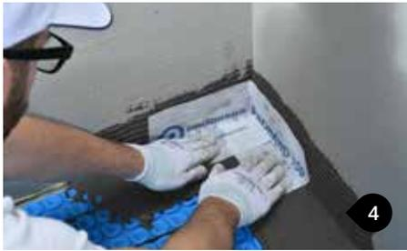
Fix **PROBAND 150/250** tape to the same type of adhesive used for tiling following the perimeter joint. Inside and outside corners can be cut from **PROBAND 150/250** tape, but pre-cut corners (**PRBI** and **PRBE**) are also available on page 19. Using a flat trowel apply strong and even pressure along **PROBAND 150/250** to ensure sealing.
