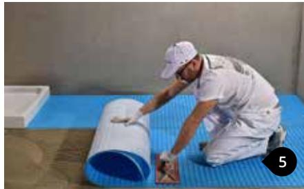
Lay the next sheet of **PRODESO HEAT MEMBRANE** taking care to align it with the previous one, without overlapping. Align the square reliefs to facilitate the installation of the heating cables.
